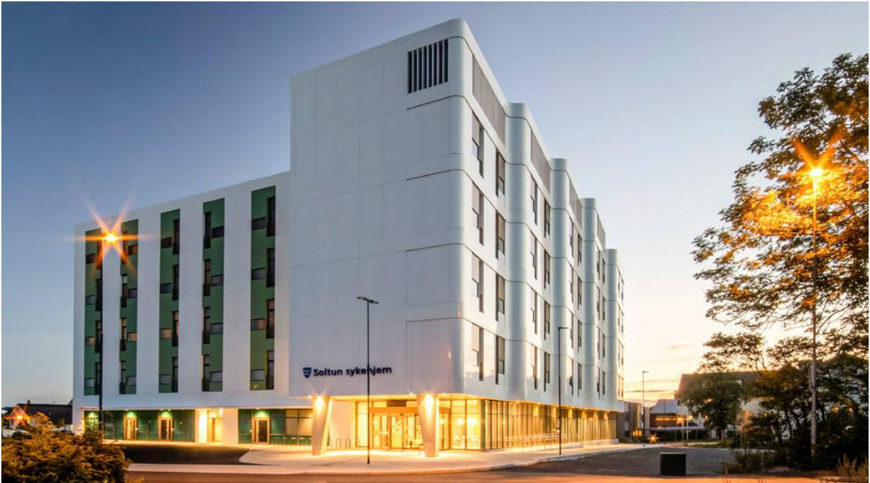
Sola Sykehjem Hospital | Sola, Norway | STB - S10
